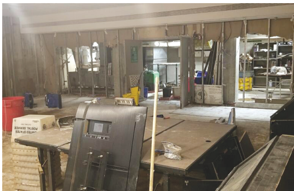
▲ The basement of 2100 Arch St. is now dry, but damaged Sheetrock and drywall will have to be demolished and replaced. Photo by Steve Rosenberg
